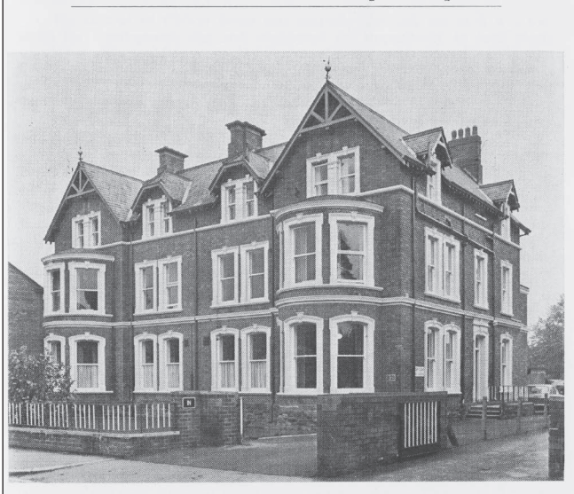
Figure 2. Alexandra Gardens Day Hospital
