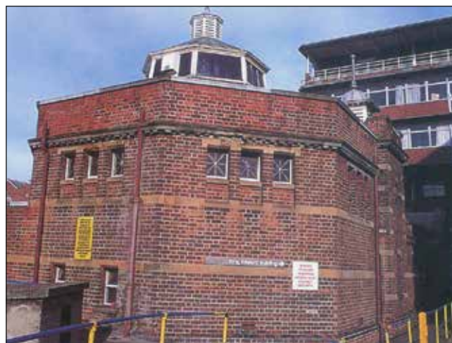
Fig 2. The old mortuary, Royal Victoria Hospital, Belfast.
