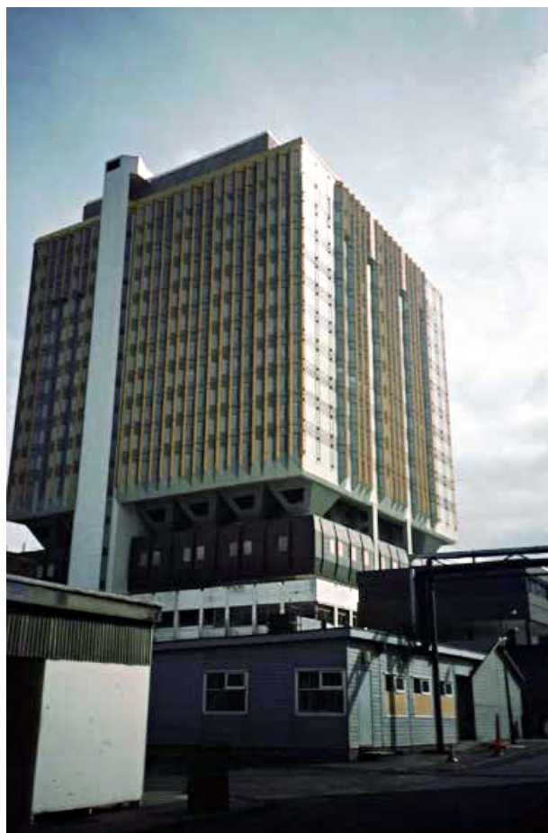
Fig 4. The completion of the West Podium Extension in 1984 (bottom right of picture just visible behind the black pipework).
