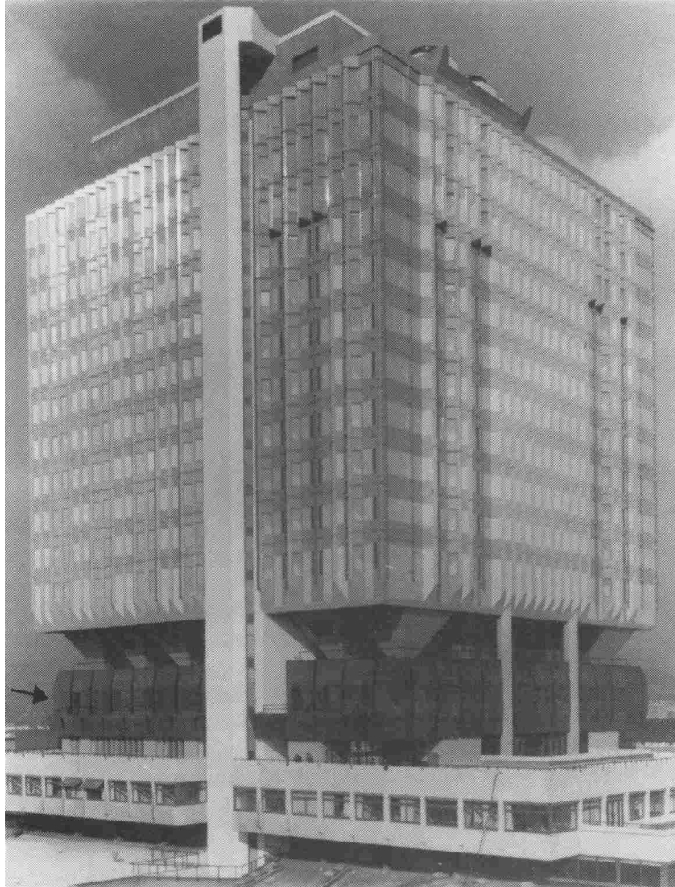
The new Belfast City Hospital, opened in 1985. The Medical School accommodation is arrowed.
